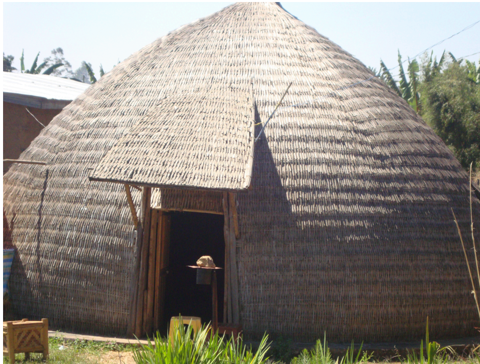
Fig. 5. Sidama traditional home made from bamboo at Arbegona, Sidama Region, southern Ethiopia. Photo by Addisu Mekonnen.
